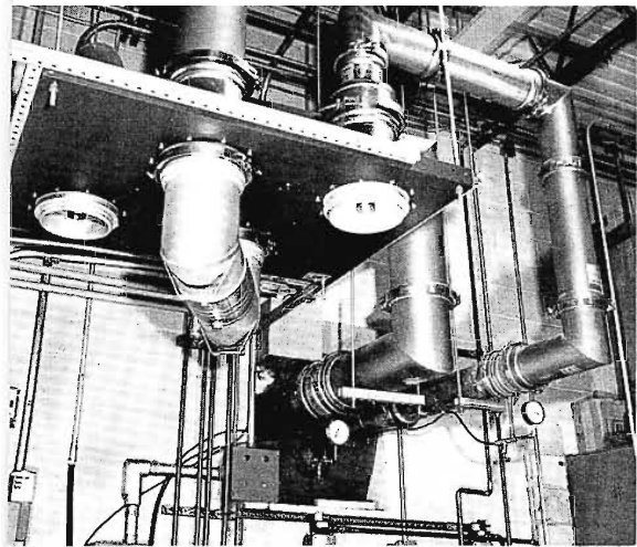
Manual coaxial patch panel for 9 \frac{3}{8} -inch transmission line to antenna.
